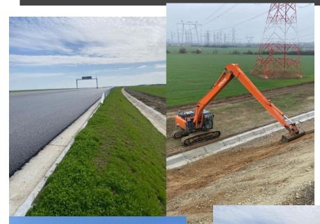
EMPLOYER: Alarko Construction WORK STATEMENT: Ring Road Project SCOPE OF WORKS:Hydro Seeding, Geocel and Top Soil Works Slope Protection with Top Soil: 600 000m2 Geocell Protection: 30 000m2 Hydroseeding Works: 600 000m2
