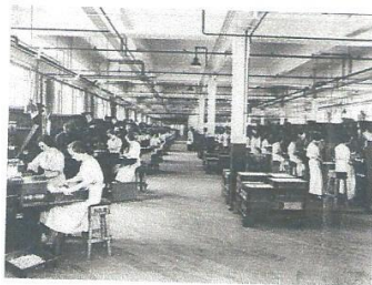
Shop floor at Nottingham factory
