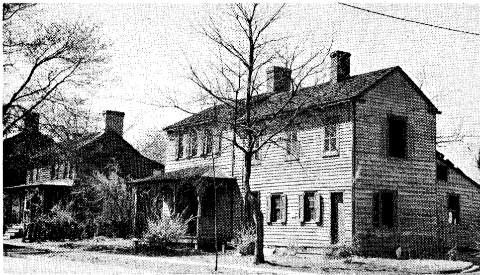
The nearer half of Miss Mary Brown's Jugtown home at 354 Nassau Street, was rented out before its last years of decay documented in this 1938 view.
