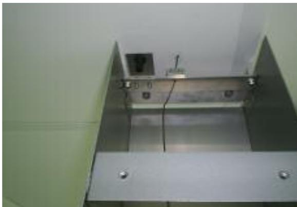
Attach plate to top of cover, make sure it is secure. At this point the cable is slack, but of course when the air on switched on, this wire will become taught.
