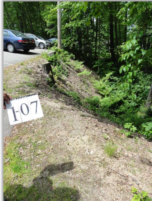
Both sites pictured above have sheet surface erosion and bare soil. The upper right picture also depicts rill surface erosion, an unstable/clogged culvert, and winter sand deposits.
