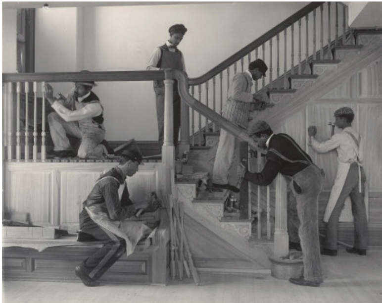
Frances Benjamin Johnston, Stairway of Treasurer's Residence, Hampton Institute, Students at Work, 1900
