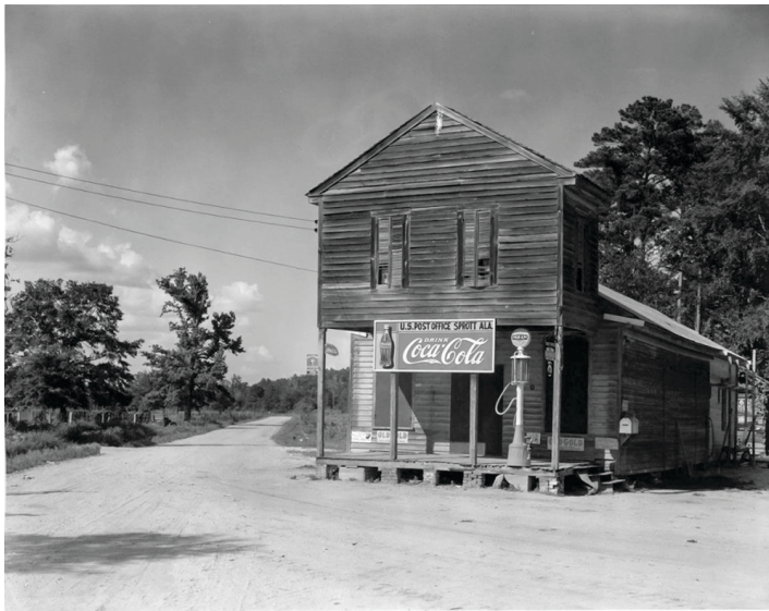
Walker Evans. Post Office, Sprott, Alabama. 1936.
