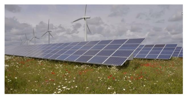
University of West London Solar PV and Solar Thermal Array linked to Ground Source Heat Pumps displaces > 3GWh of gas per year
