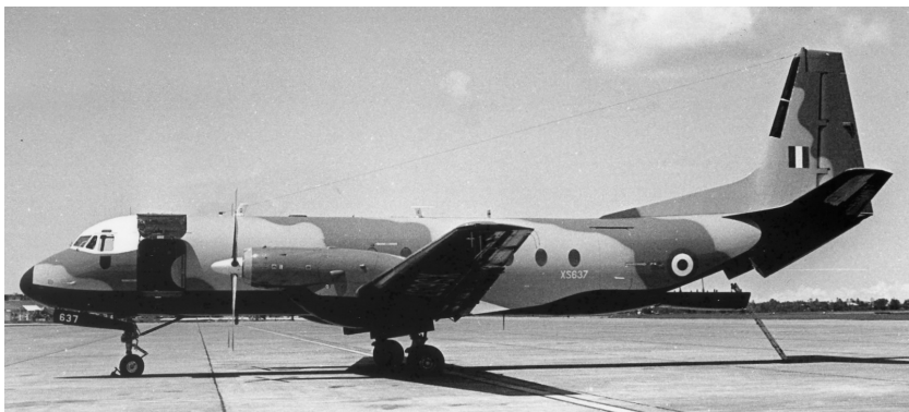
The Andover had a kneeling undercarriage in order to reduce the gradient of the access ramp.
