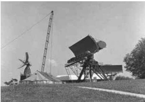
Bukit Gombak with its Marconi search radar and Plessey height finder.
