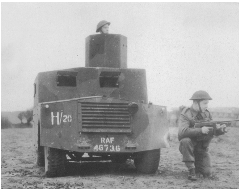
A Beaverette Mk I. The Mk III had a more substantial turret mounting, for AA purposes, a pair of 0.303" Vickers 'K's.
