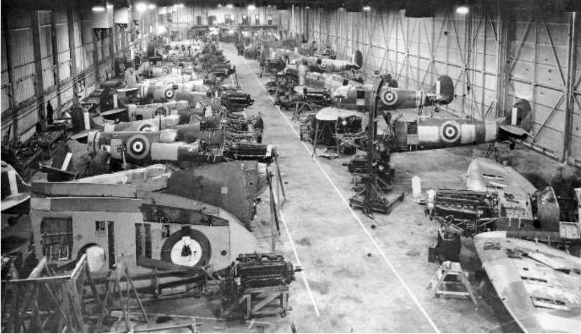
Salvaged Spitfires being rebuilt in a CRO plant circa 1941.
