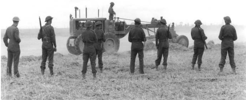
Heavy plant being used to level an airstrip in Normandy.
