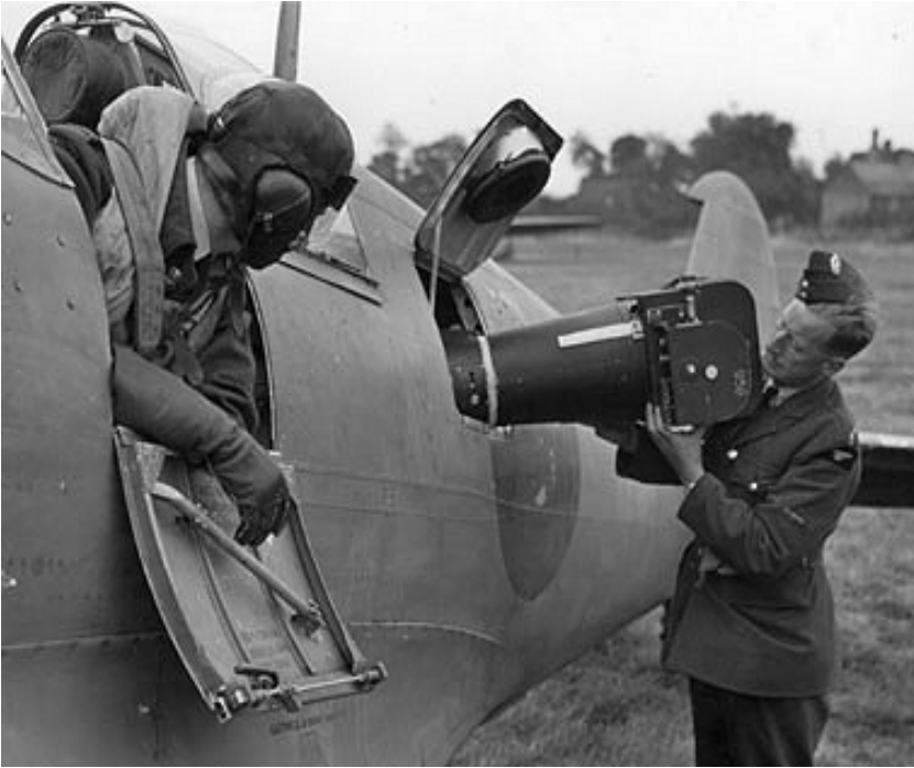
An airmen loading a camera, in this case an F8, into a Spitfire.
