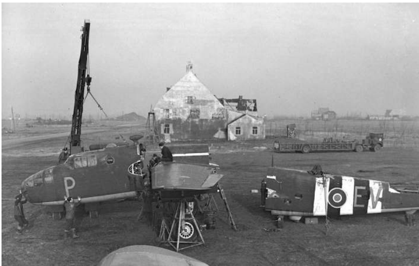
A damaged Mitchell, FW161 of No 180 Sqn being, surgically dissected prior to loading onto a 'Queen Mary'.
