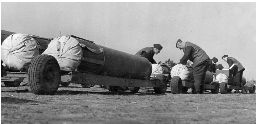
Parachute-retarded mines being fused.
