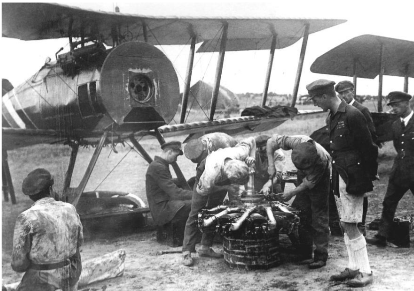
Mechanics resolving a problem with the Bentley BR2 engine of one of No 203 Sqn's Nightjars.
