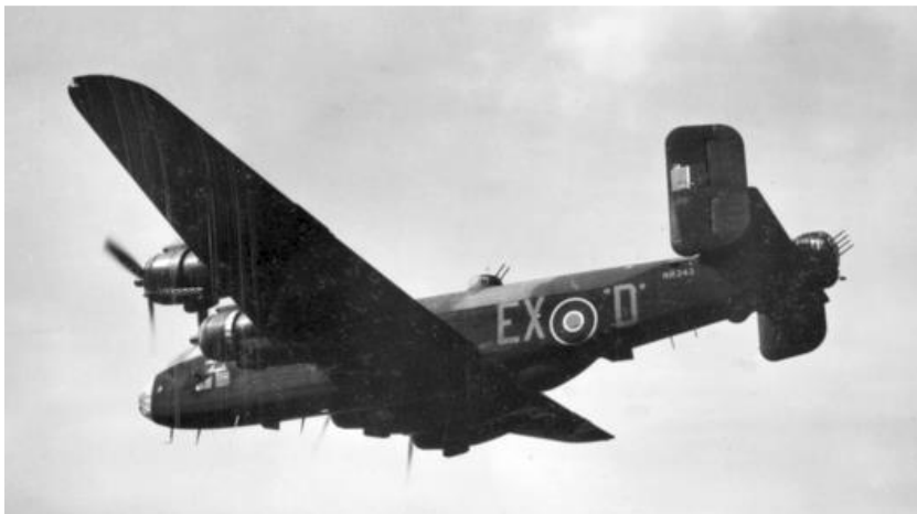
A Halifax of No 199 Sqn with a selection of (barely discernible) Mandrel blade aerals on the lower fuselage.
