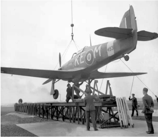
An MSFU Hurricane, Z4935, being prepared for a practice launch at Speke with a number of, still to be loaded, rockets at the rear of the catapult. (IWM CH 15390).
