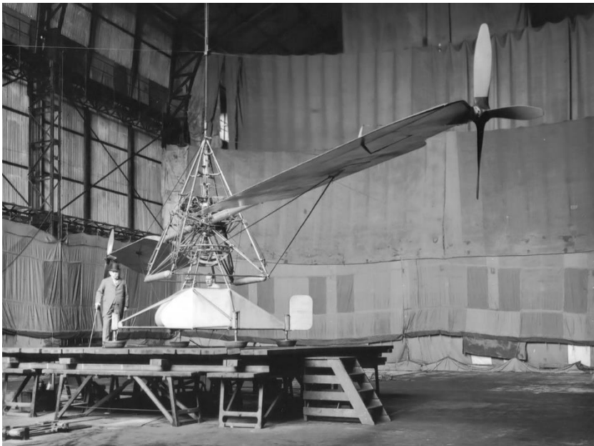
The Brennan helicopter with its unique prop-driven rotor.
