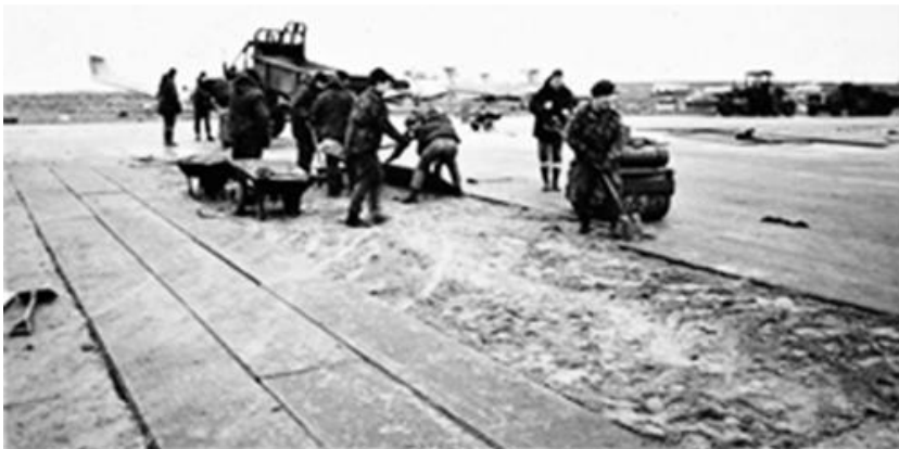
Stanley's runway being repaired and extended with US-supplied AM2 panels.
