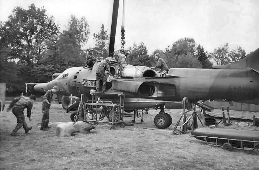
Extreme engineering – an engine change in the field. ('21zebra')
