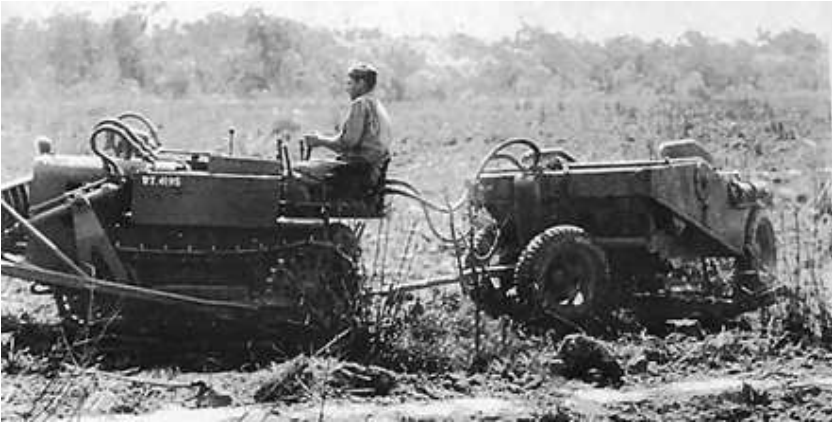
The Clark CA-1 Tractor and LaPlant-Choate CAB-1 pan scraper that were instrumental in levelling an airstrip at Broadway.
