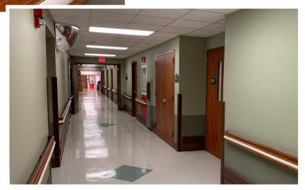
Glenwood is an older facility, with plaster walls that, over the years, had been weakened by cracks, gouges and tears from rolling beds and service carts. In some high traffic areas, the same portions of the wall surface had been patched four and five times.
