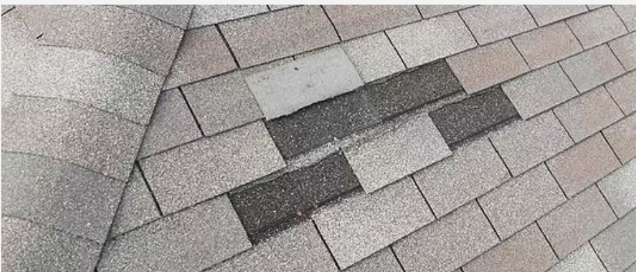
MISSING SHINGLES
