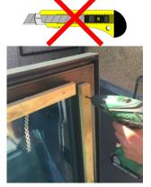
2 - Remove any loose debris from the upstand and apply a generous bead of the relevant sealant (see above) to eliminate any drafts.
