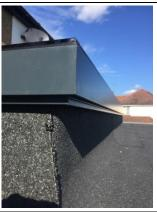
4 - Centralise the inside of the roof with the internal upstand, this will allow the plasterboard to fit neatly into the plasterboard pocket.
