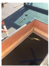
3 - Make sure the roof has an overhang all round, to allow water to discharge.
