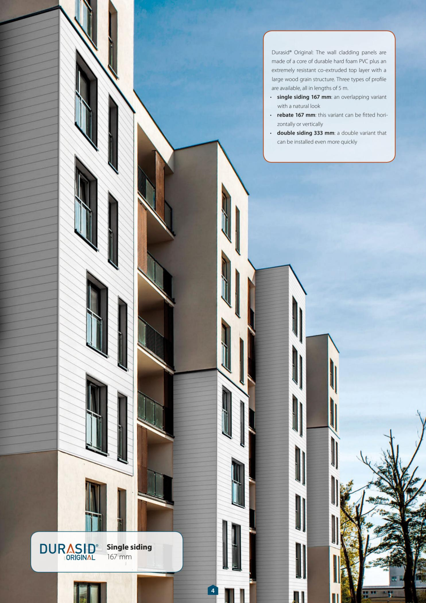
Durasid® Original: The wall cladding panels are made of a core of durable hard foam PVC plus an extremely resistant co-extruded top layer with a large wood grain structure. Three types of profile are available, all in lengths of 5 m.
