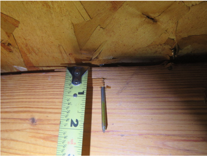
Roof Deck Attachment
