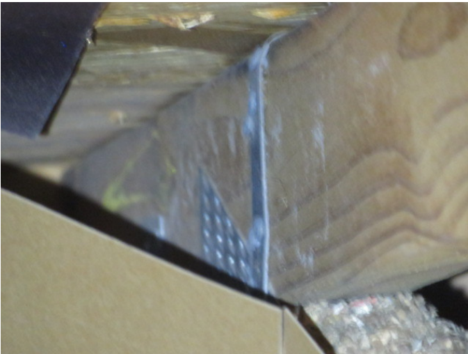
Roof to Wall Attachment
