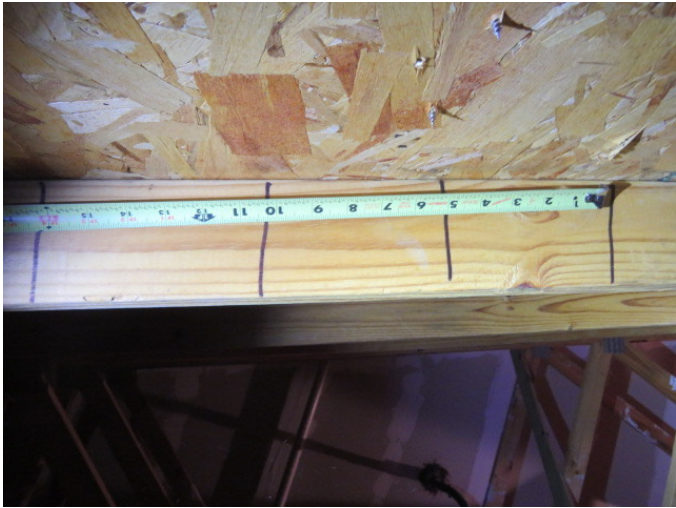
Roof Deck Attachment
