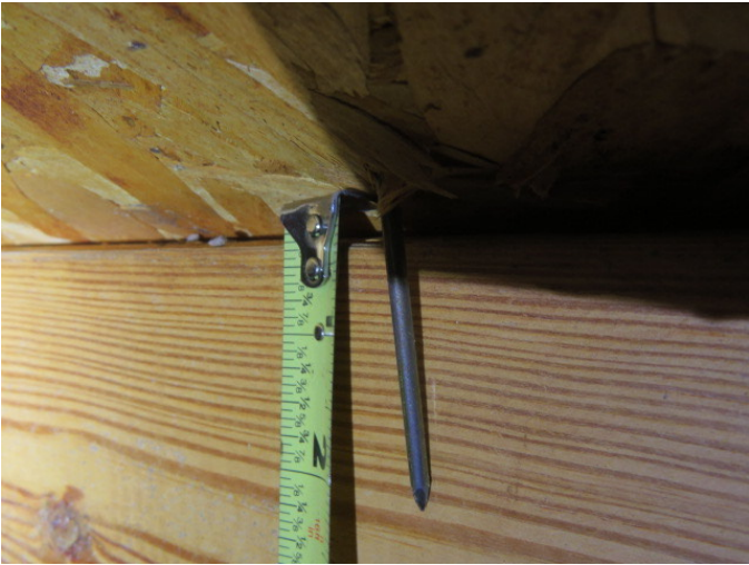
Roof Deck Attachment
