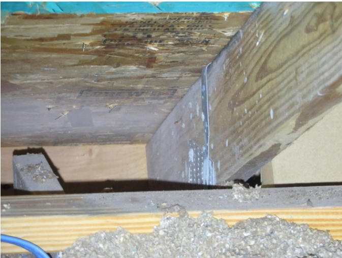
Roof to Wall Attachment
