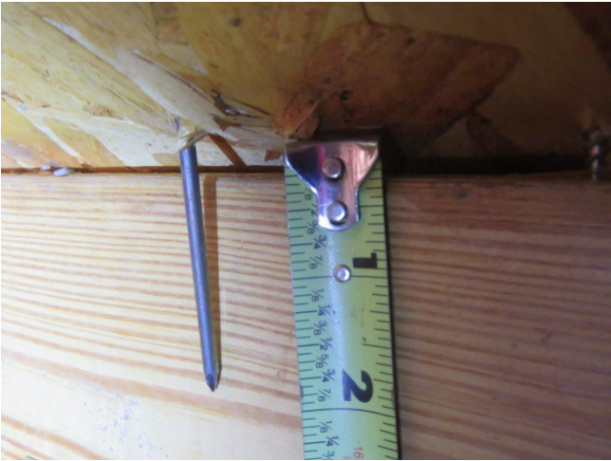
Roof Deck Attachment
