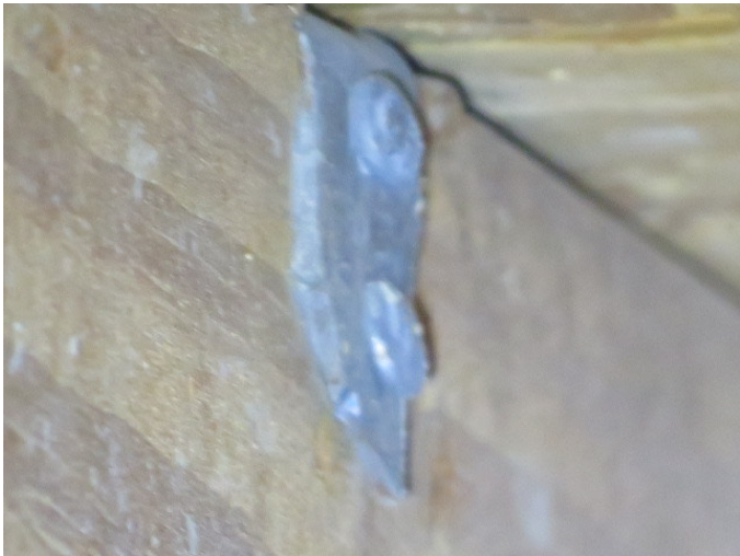
Roof to Wall Attachment
