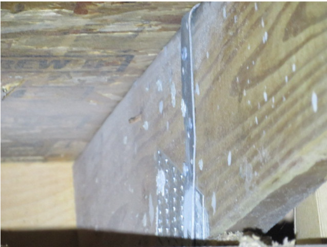
Roof to Wall Attachment
