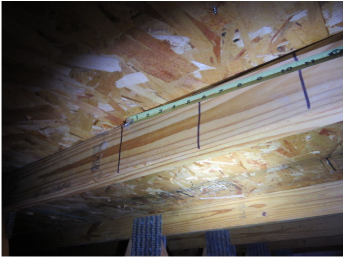
Roof Deck Attachment
