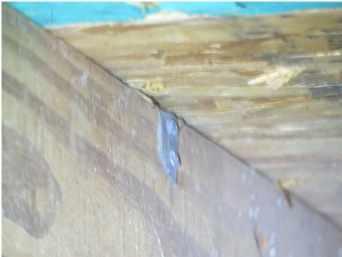
Roof to Wall Attachment
