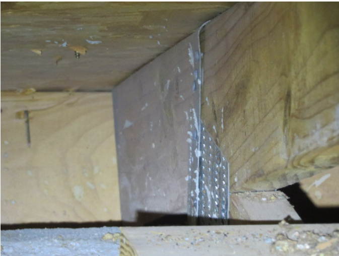
Roof to Wall Attachment
