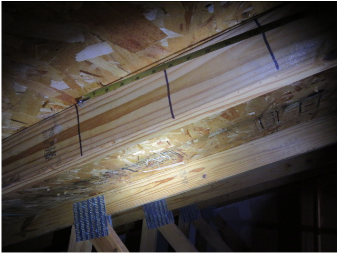
Roof Deck Attachment
