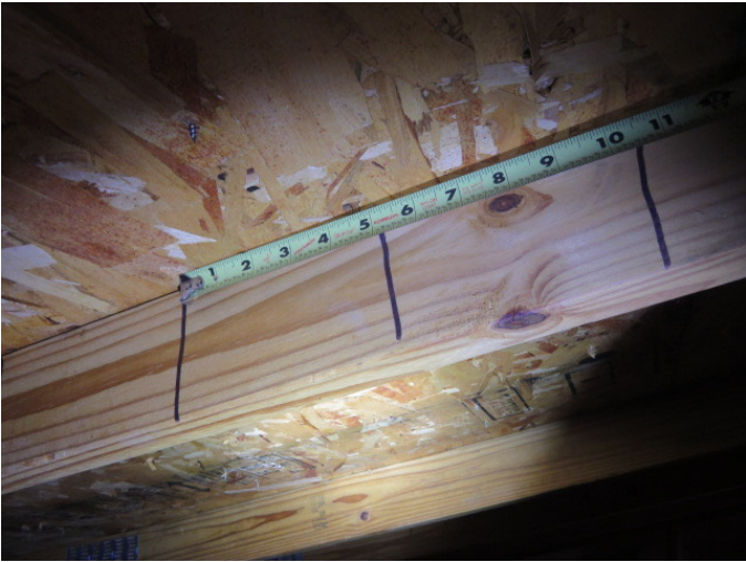
Roof Deck Attachment
