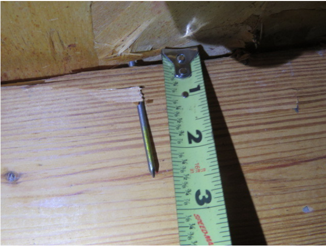
Roof Deck Attachment
