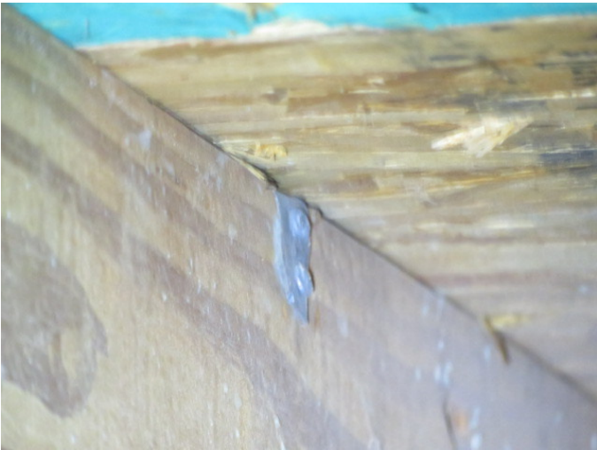
Roof to Wall Attachment
