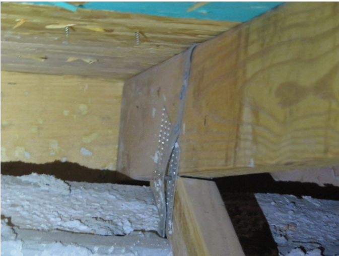
Roof to Wall Attachment
