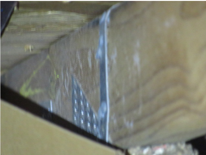
Roof to Wall Attachment
