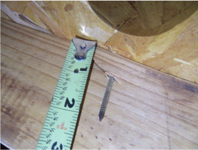
Roof Deck Attachment
