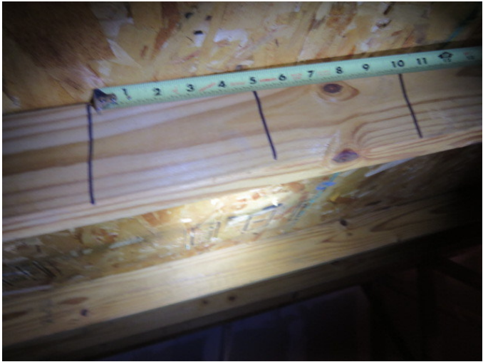
Roof Deck Attachment
