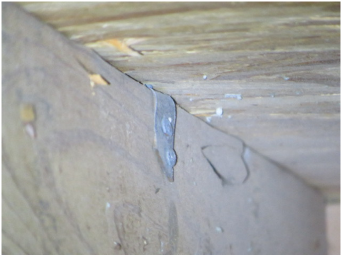
Roof to Wall Attachment
