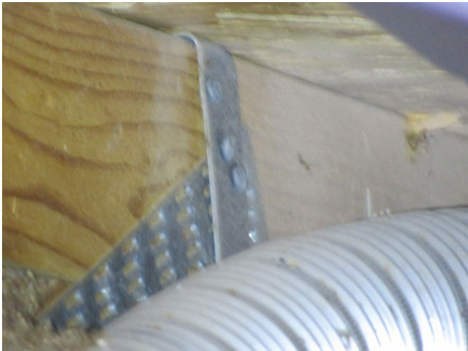
Roof to Wall Attachment
