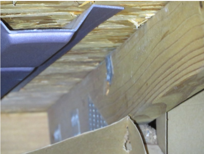
Roof to Wall Attachment
