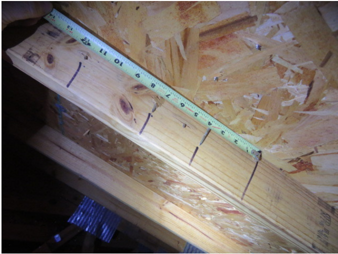
Roof Deck Attachment
