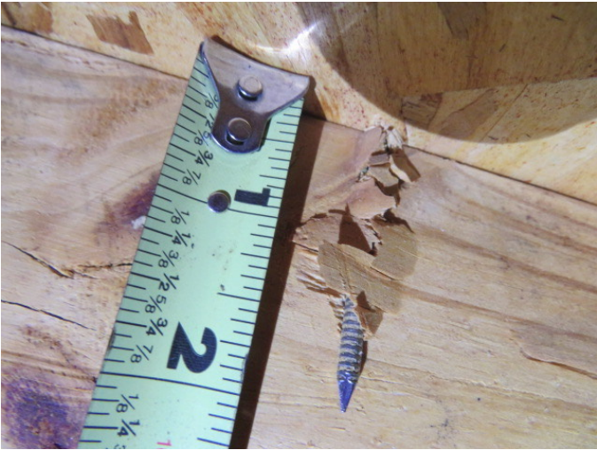
Roof Deck Attachment
