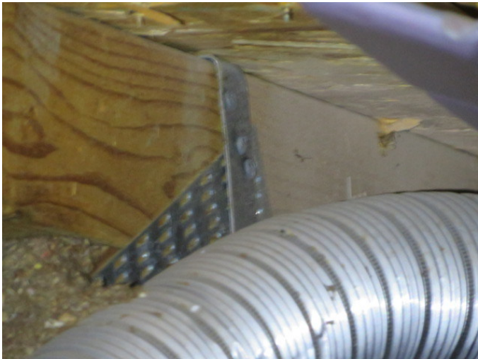
Roof to Wall Attachment
