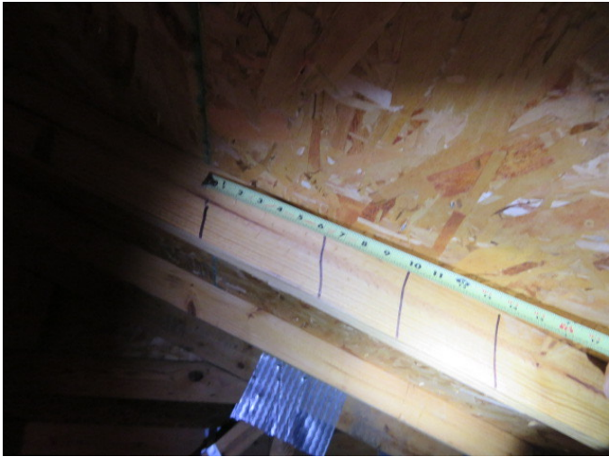
Roof Deck Attachment
