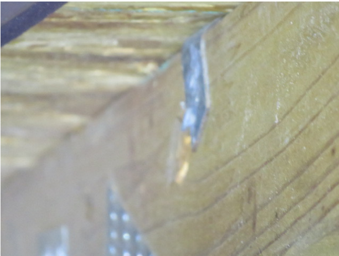
Roof to Wall Attachment
