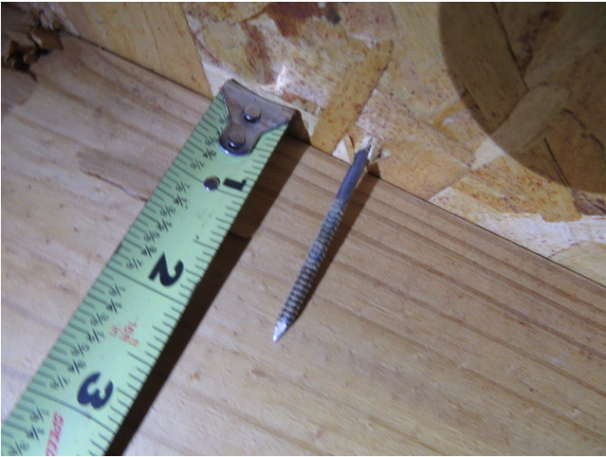
Roof Deck Attachment
