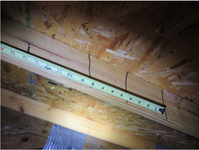
Roof Deck Attachment
