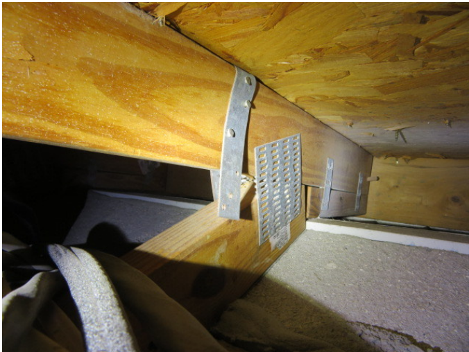
Roof to Wall Attachment
