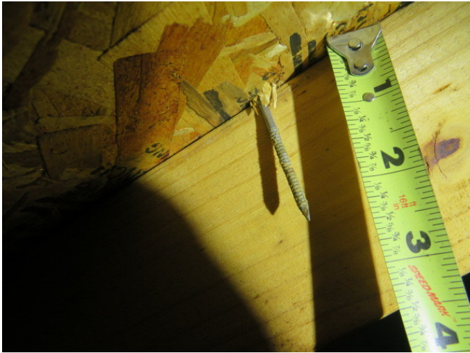
Roof Deck Attachment
