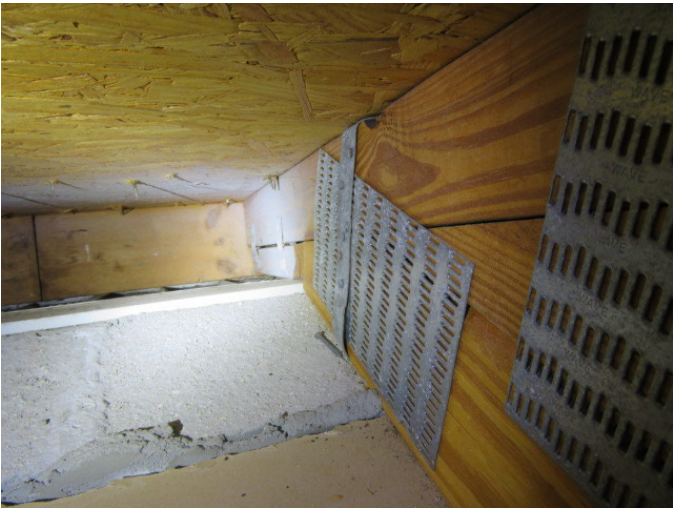
Roof to Wall Attachment
