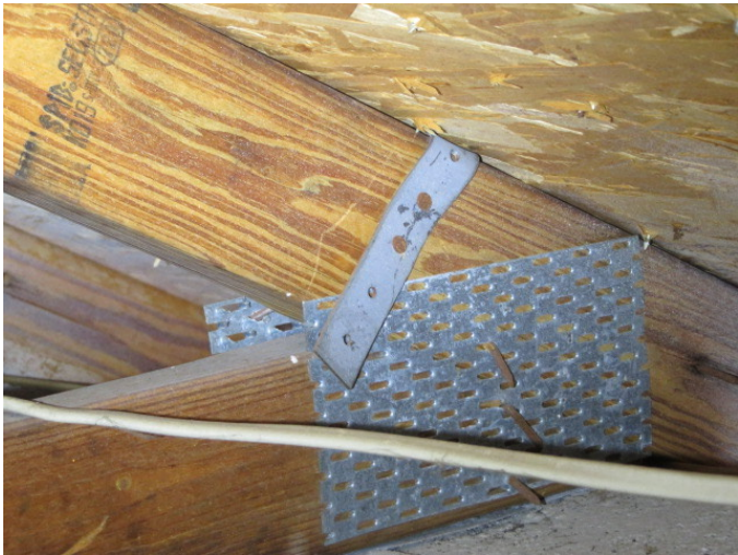
Roof to Wall Attachment
