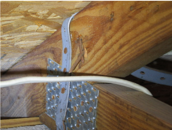
Roof to Wall Attachment
