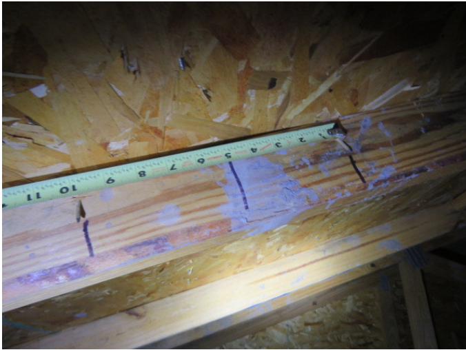
Roof Deck Attachment
