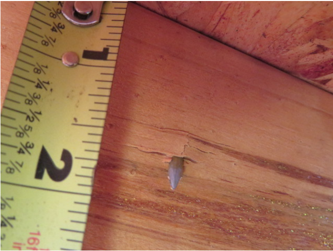
Roof Deck Attachment
