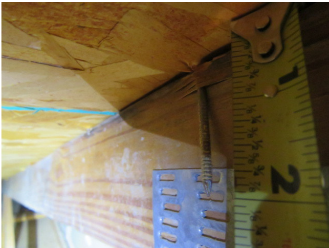
Roof Deck Attachment
