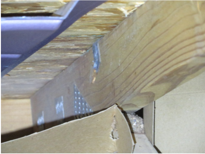
Roof to Wall Attachment
