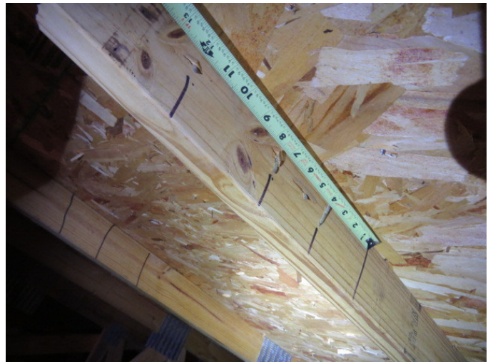
Roof Deck Attachment
