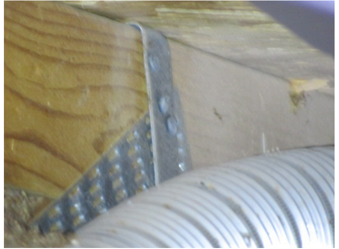
Roof to Wall Attachment
