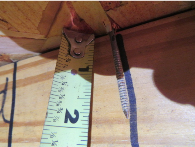
Roof Deck Attachment
