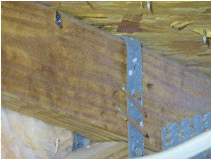
Roof to Wall Attachment
