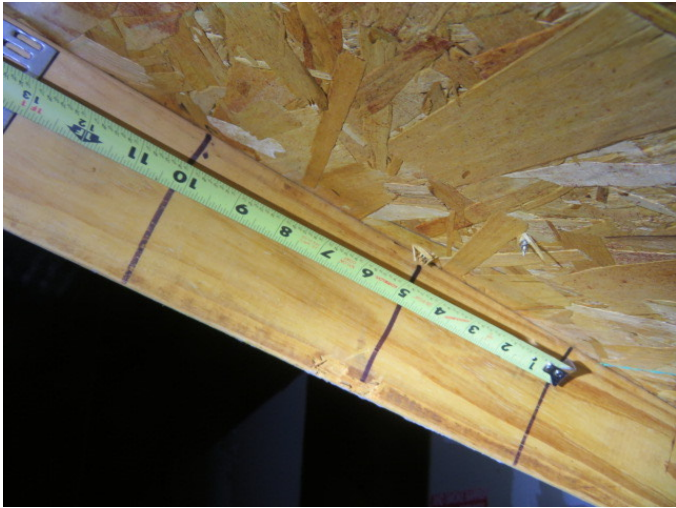
Roof Deck Attachment
