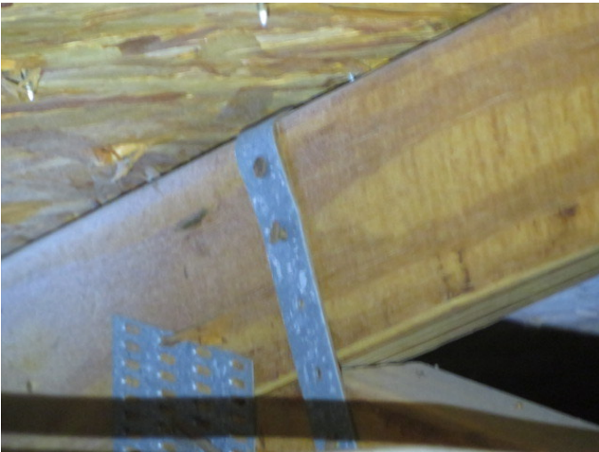
Roof to Wall Attachment
