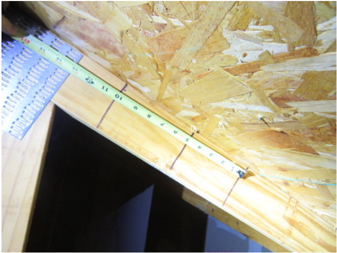
Roof Deck Attachment
