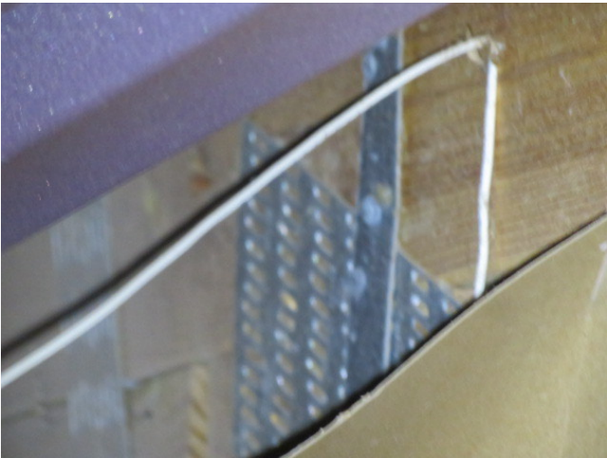
Roof to Wall Attachment
