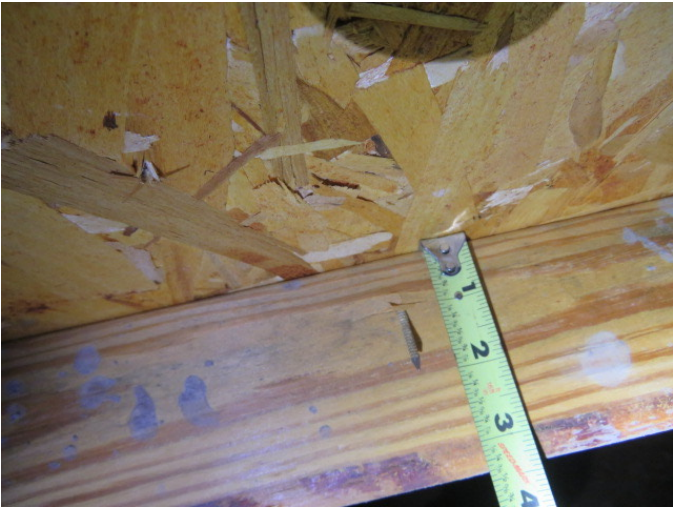
Roof Deck Attachment
