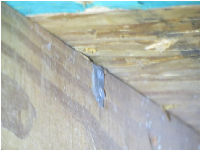
Roof to Wall Attachment
