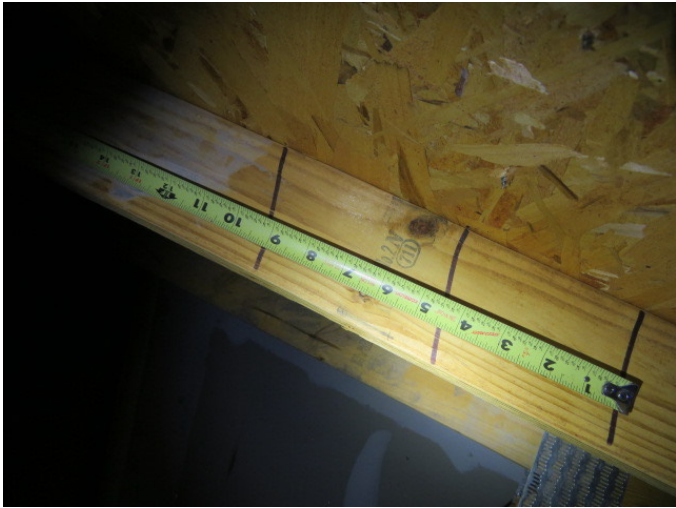
Roof Deck Attachment
