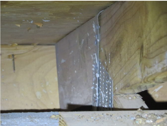
Roof to Wall Attachment
