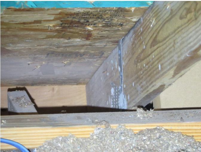
Roof to Wall Attachment
