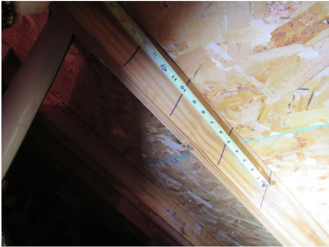
Roof Deck Attachment
