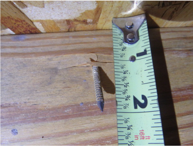
Roof Deck Attachment
