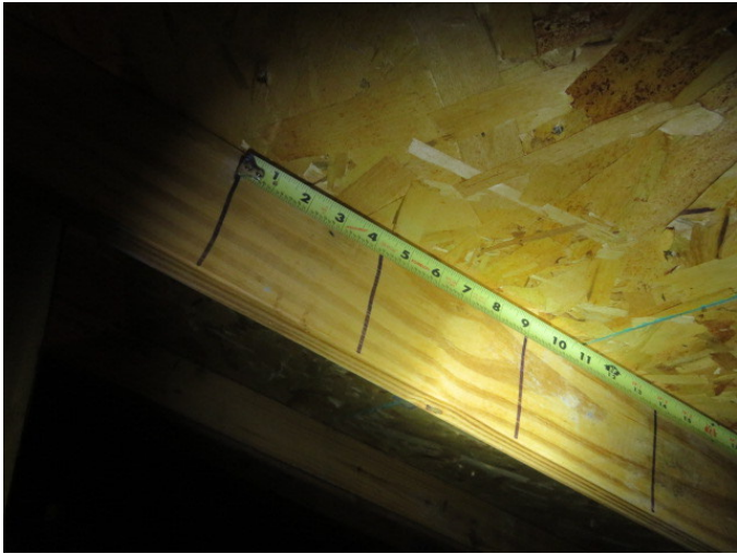
Roof Deck Attachment
