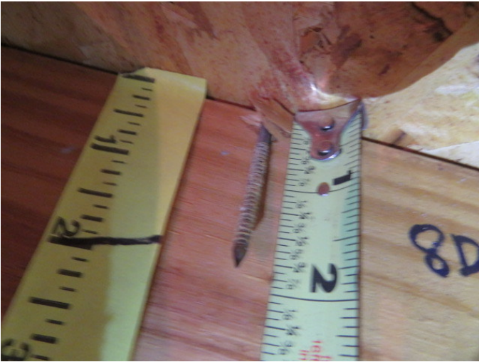
Roof Deck Attachment
