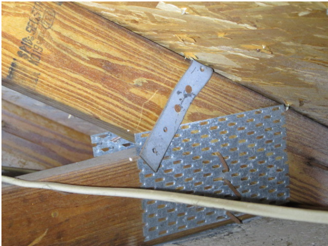
Roof to Wall Attachment
