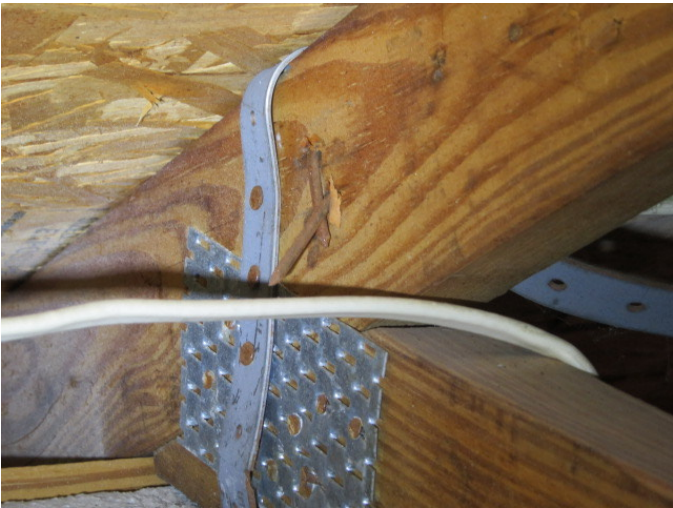
Roof to Wall Attachment
