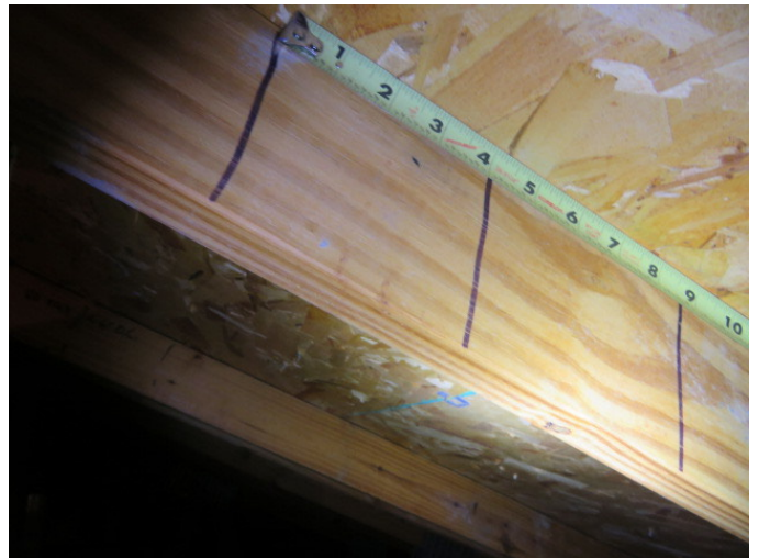
Roof Deck Attachment
