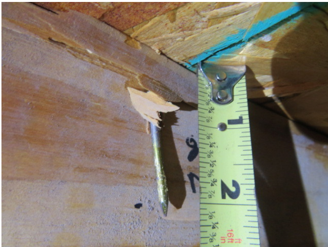
Roof Deck Attachment
