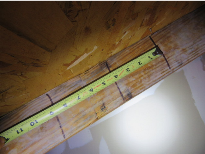
Roof Deck Attachment
