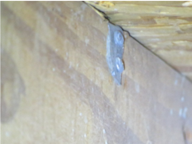
Roof to Wall Attachment
