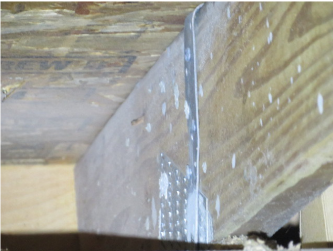
Roof to Wall Attachment
