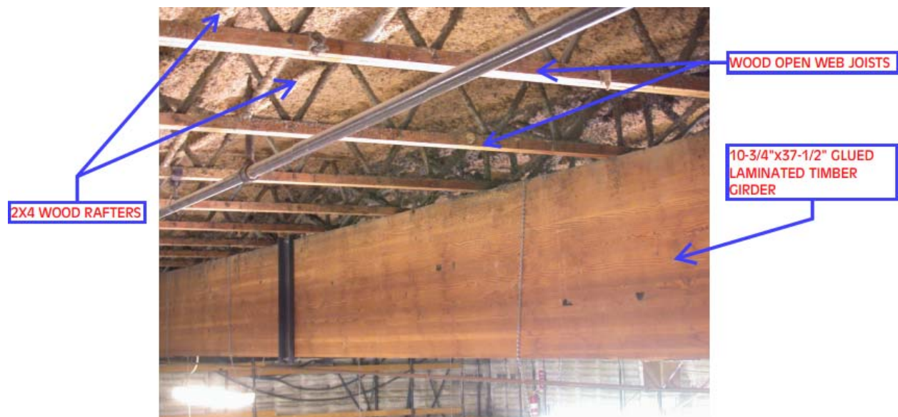
Figure 1: Existing Roof Structure (2x4 Rafters Are Covered by Fireproofing)
