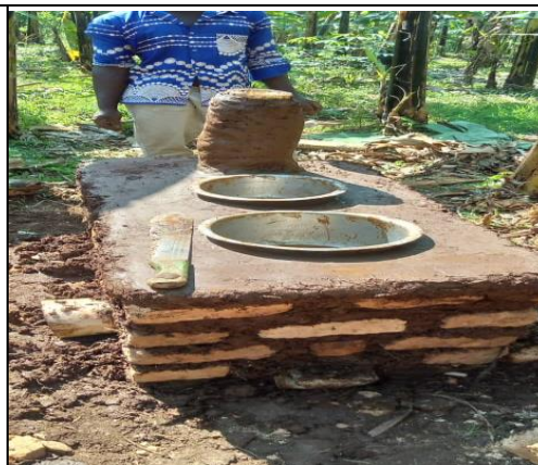
Rwambu Parish in Kijongo. A complete Biomass cook stove constructed by members
