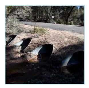
Culverts are corrugated metal piping. Please note that the estimated cost is for replacement of the existing culverts with corrugated PVC piping and does not consider any need for future installation of new culverts as it is assumed the roads/culvert system was designed appropriately and with adequate drainage. Should new culverts be installed at a future date they can then be added to updates to this reserve study.
