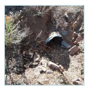
Culverts are (corrugated metal/corrugated PVC) piping. Please note that the estimated cost is for replacement of the existing culverts with corrugated PVC piping and does not consider any need for future installation of new culverts as it is assumed the roads/culvert system was designed appropriately and with adequate drainage. Should new culverts be installed at a future date they can then be added to updates to this reserve study.
