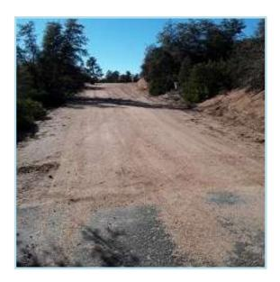
Appears to be deteriorating at a rate typical of its age. As routine maintenance, keep surface clean, ensure that drains are clean and free flowing, repair cracks and clean oils stains promptly. Best to plan for eventual intervals of resurfacing (overlay).
