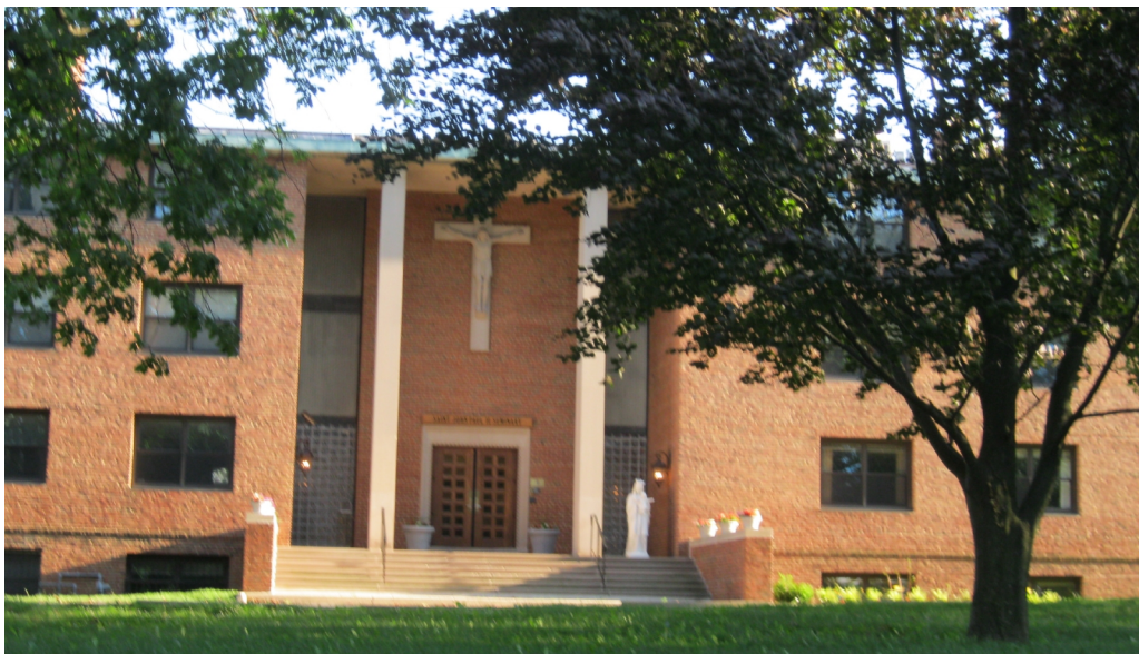
The new Atonement Seminary building was opened in 1957 and served our Friars of the Atonement until 1999. Today the seminary building has become the Saint John Paul II Seminary for the Archdiocese of Washington, D.C. Note the statue of Our Lady of the Atonement still stands on the front step!
