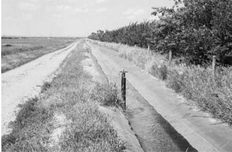
**Fig. 13.3** An asphalt-lined irrigation channel in Victoria.
