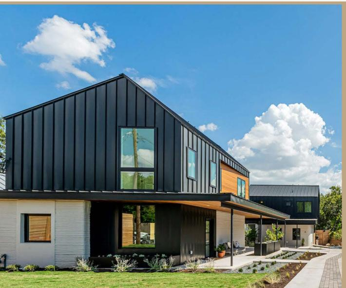
ICON'S 3D PROPRIETARY printing technology produces resilient, energy-efficient homes faster than conventional construction methods with less waste and more design freedom - keeping construction projects on schedule with huge savings
