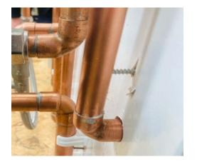
The pipes were secured using screws through the plywood
