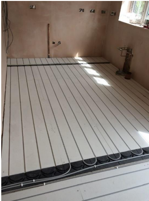
Heavyweight Overlay Installation
