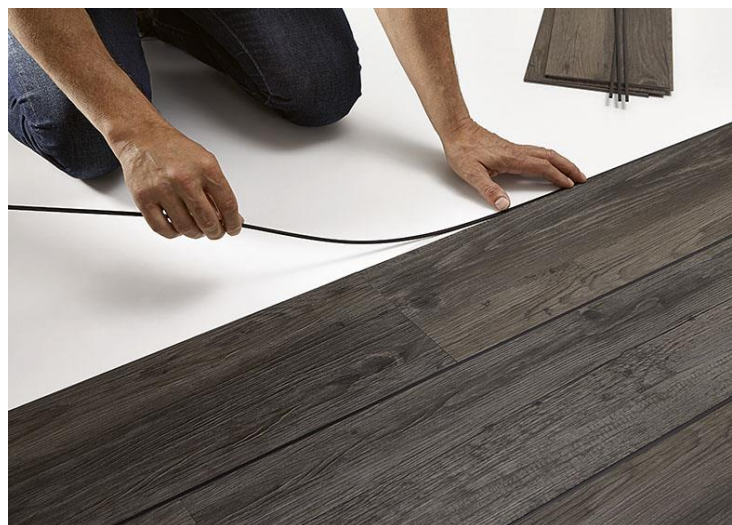
Installation of luxury vinyl tile (LVT)
