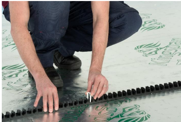
Clipping the rails to the insulation
