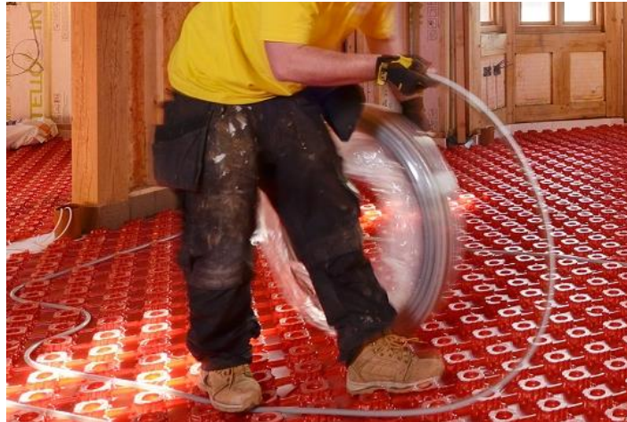
Laying the pipe
