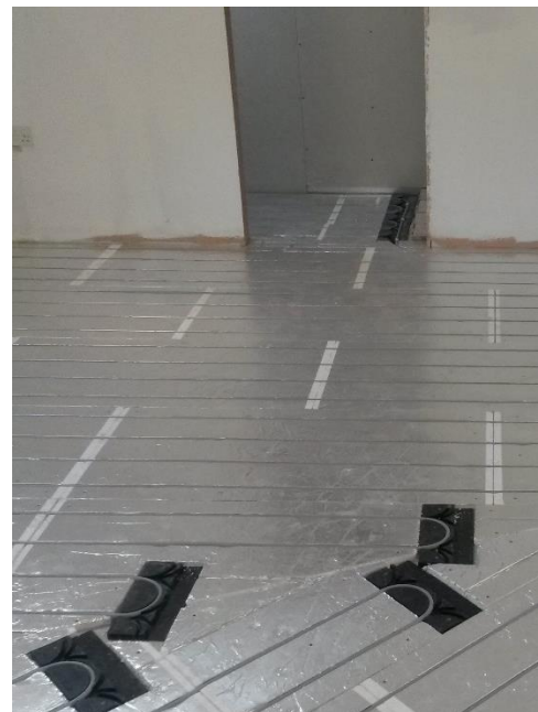
Lightweight Overlay Installation
