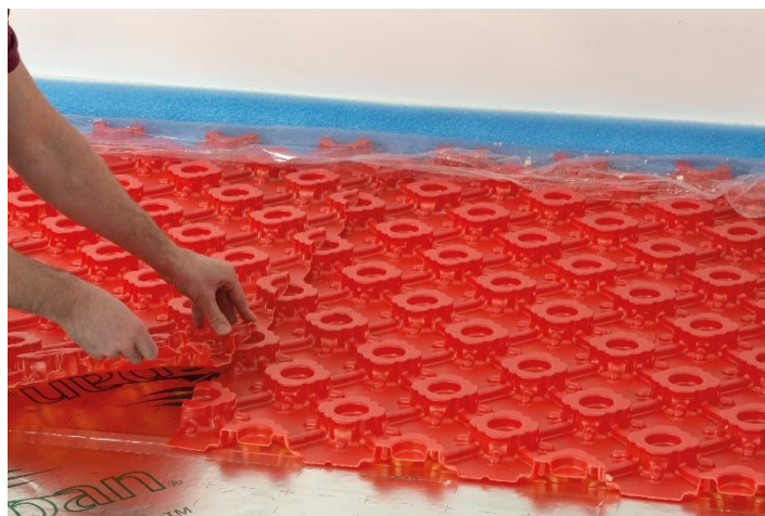
Laying the panels
