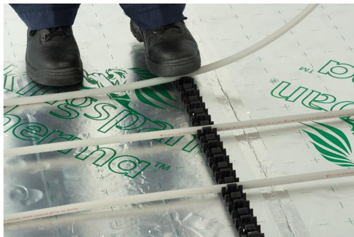
Clipping the pipe into the rails
