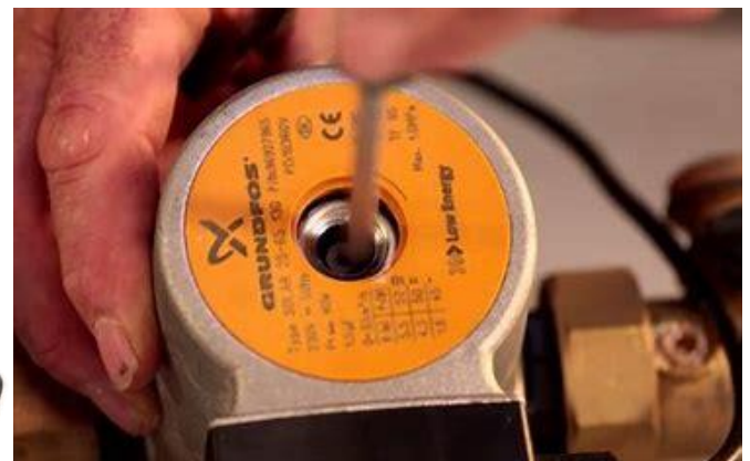
Above is an unprofessional situation the pump screw is above the electrical connections so ideally the head needs rotating
