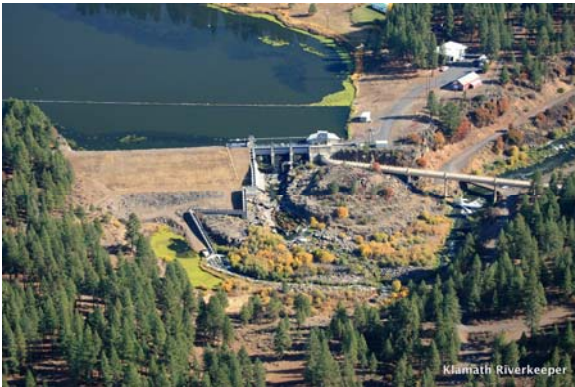
Figure 1. J.C. Boyle Dam.
