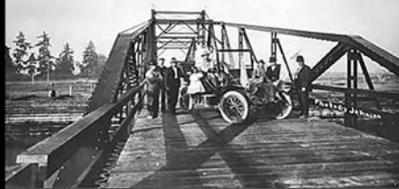
1909 Swing Bridge to Camano Island
